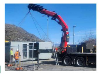
An above-ground diesel tank has been installed on the airfield as part of our resilience plan. It holds enough fuel to keep the terminal running for a few weeks in the event of a major emergency, such as a large earthquake.
